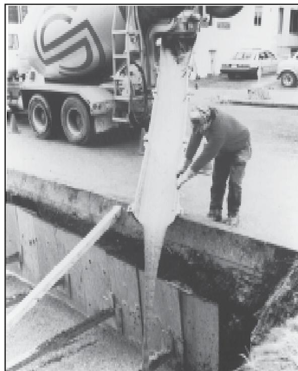
Higher strength structural fills can be designed for a specific required strength. Compressive strength of 50 to 100 psi (0.3 to 0.7 MPa) provides an allowable bearing capacity similar to well-compacted soil.
